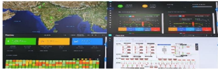
Centralised Control Room for Proactive Asset Management
